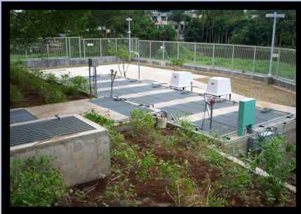
JET INSTALLATION IN RANGOON, BURMA WITH EFFLUENT BEING USED FOR IRRIGATION
