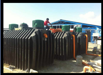
PORTABLE STP INSTALLED IN MARINA BAY PROJECT JET 500-800 PLT 20 CUBIC METER
